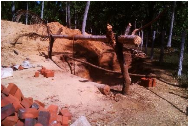
The well under construction
